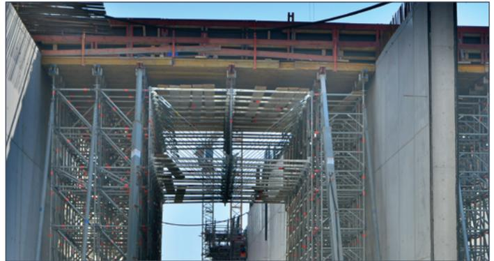
▶ Bridging structure/passageway in shoring scaffolding using the Allround FW System.
