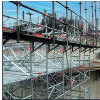
▶ Side protection at the edge of a slab.
