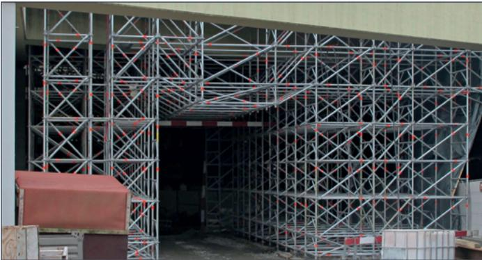
▶ Bridging structure/passageway in shoring scaffolding using standard Allround Scaffolding material.
