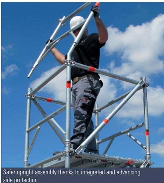
Safer upright assembly thanks to integrated and advancing side protection
