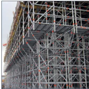
▶ Attachment of bracket deck surfaces at edge.
